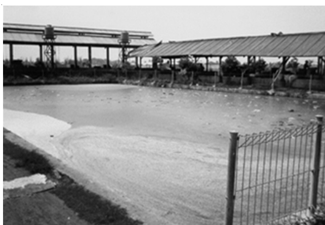
Fig. 6. Wastewater treatment of small tofu industry at Semanan, Jakarta Barat
